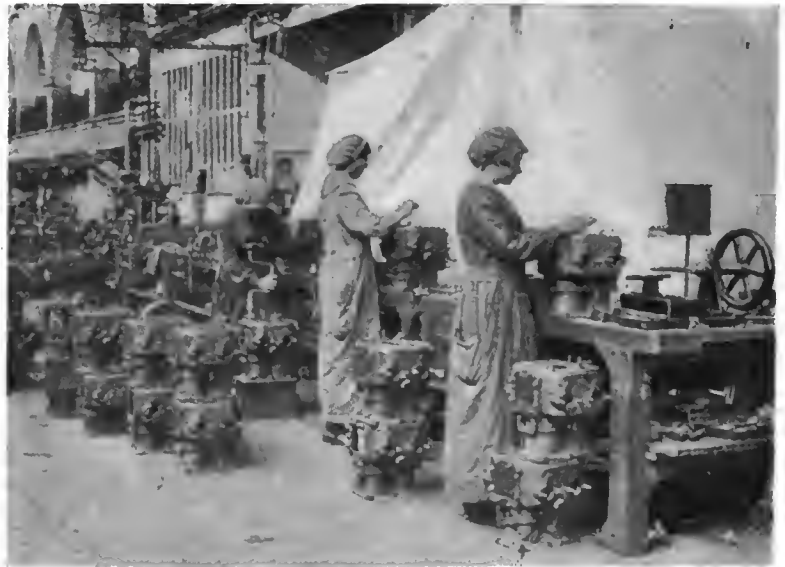
Women operators doing what was formerly men's work, shaping small parts and grinding in valves of truck engines
